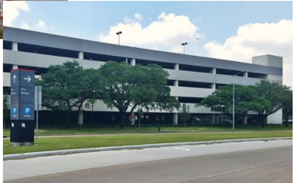
Elgin Street Garage
