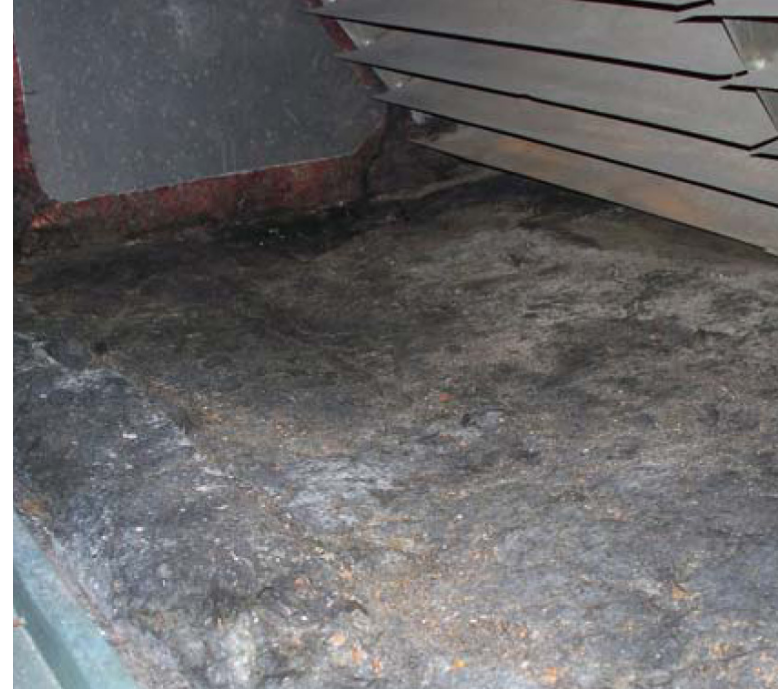
Fraying ductliner
