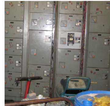
E3: Modified Federal Pacific Motor Control Center Bucket
