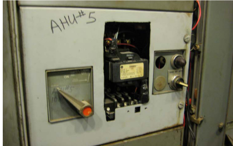
E3: Modified Federal Pacific Motor Control Center Bucket
