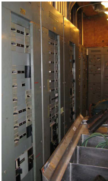
E4, 5, 6: Example of Storage in violation of NEC working clearance requirements.
