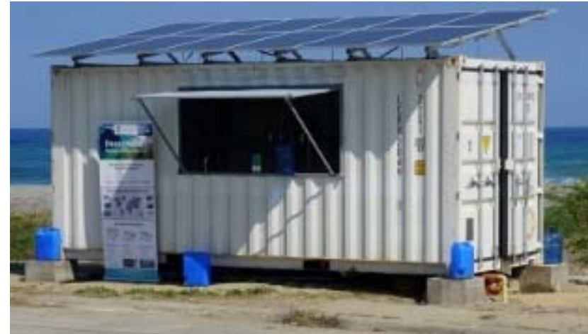
11 m 3 /d PV powered RO system from Elemental Water Makers, Philippines
